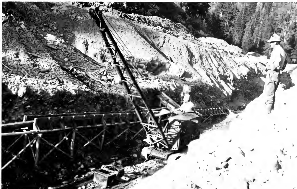
Photo 70. Steam Dragline Operation, Trinity River District. The photo was taken at Coffee Creek, Trinity County, in the 1920s. Photo by C. V. Averill.
