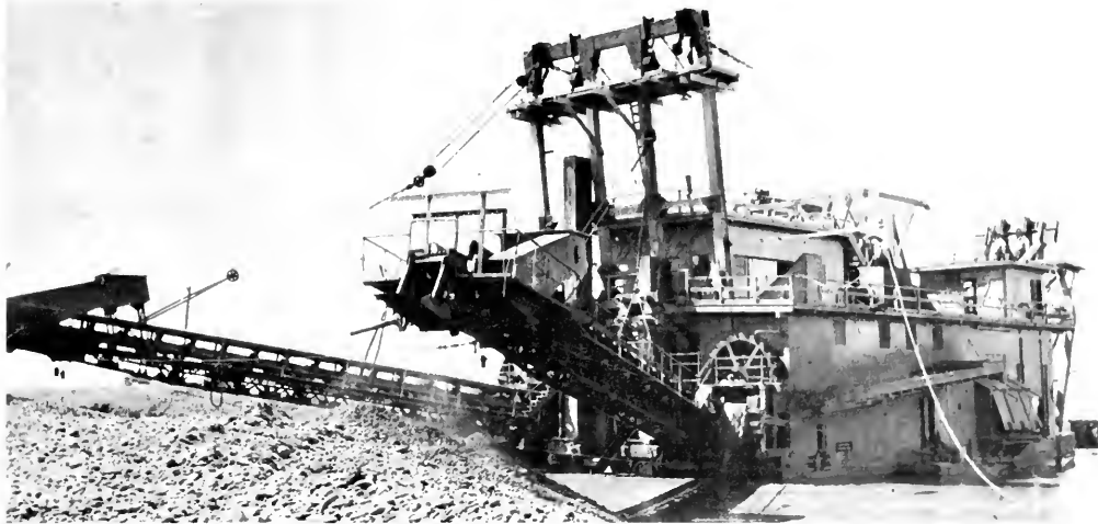
Photo 19. Natomas Company Dredge No. 2, Folsom District. This 1921 view of the dredge, in Sacramento County, shows the double stackers and sand wheel. Photo by C. A. Waring.
