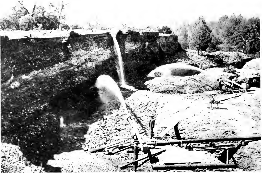
Photo 67. Princess Hydraulic Mine, Shasta County. The monitors are undercutting a bank of auriferous gravel. The photo was taken in about 1900. Photo courtesy of Adele Kiessling.
