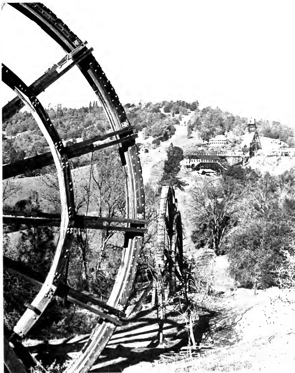
Photo 34. Kennedy Mine, Recent View. This view, to the north, shows the tailings wheels, headframe and remaining buildings at
