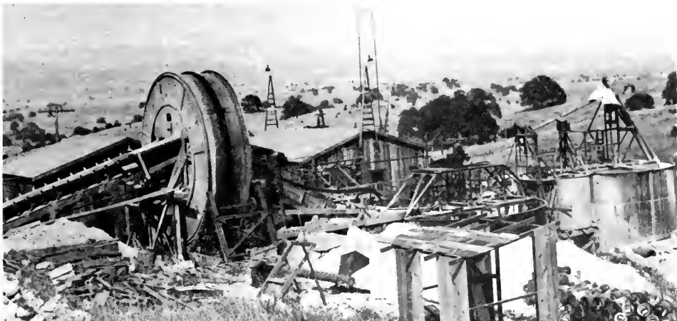
Photo 29. Doss (Ginaca) Mine, Hornitos District. This 1934 view of the Mariposa County mine shows a Hadsel mill, at left. Photo by Ralph Baverstock, from collection of Dr. Horace Parker.
