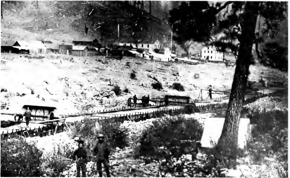
Photo 27. Mining Operations, Grizzly Flat District. The photo was taken in the 1850s. Photo courtesy of Bancroft Library.
