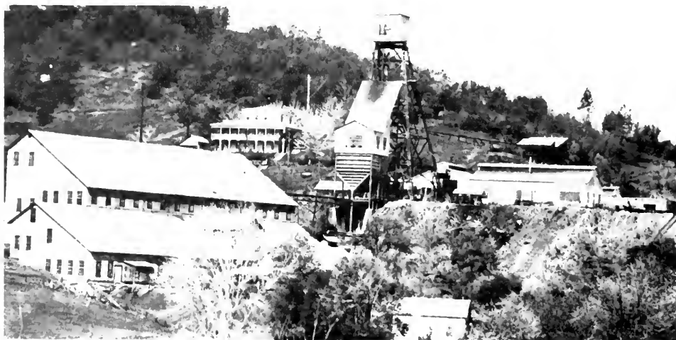
Photo 33. Kennedy Mine and Mill, Jackson-Plymouth District. This view, looking north, shows the Amador County mine and 100-stamp mill in about 1936. At that time, the Kennedy was the deepest mine
