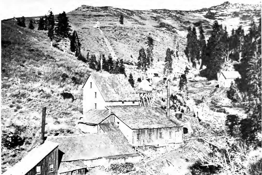
Photo 66. Bully Choop Mine, Bully Choop District. This view, in about 1900, shows the 30-stamp mill and tramway at the mine, in
