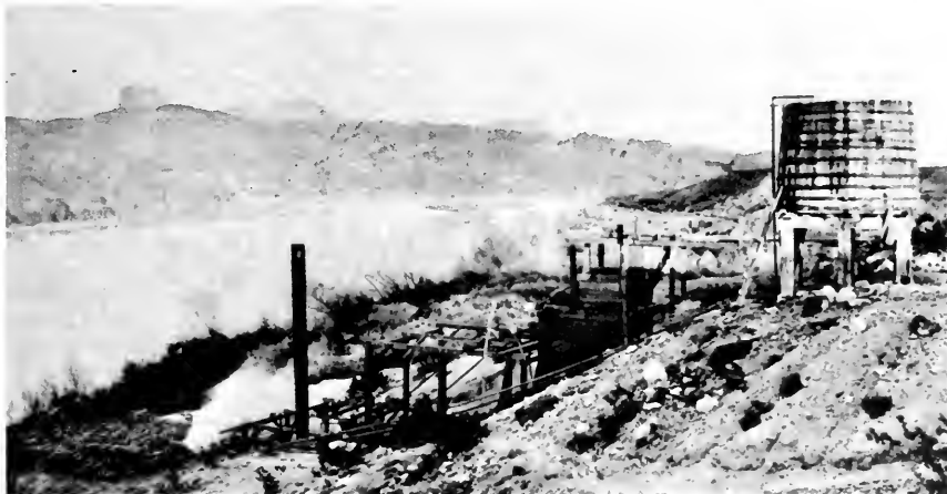
Photo B1. Gold Concentrating Mill, Colorado River. Steam powered this mill on the Arizona side of the Colorado River in the early 1900s. Picacho Peak is in the left background.
