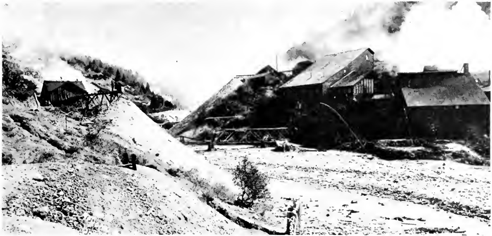
Photo 50. Providence Mine, Nevada City District. This 1893 view of the mine, in Nevada County, looks southeast. The Champion mine is at left, Deer Creek in the foreground.
