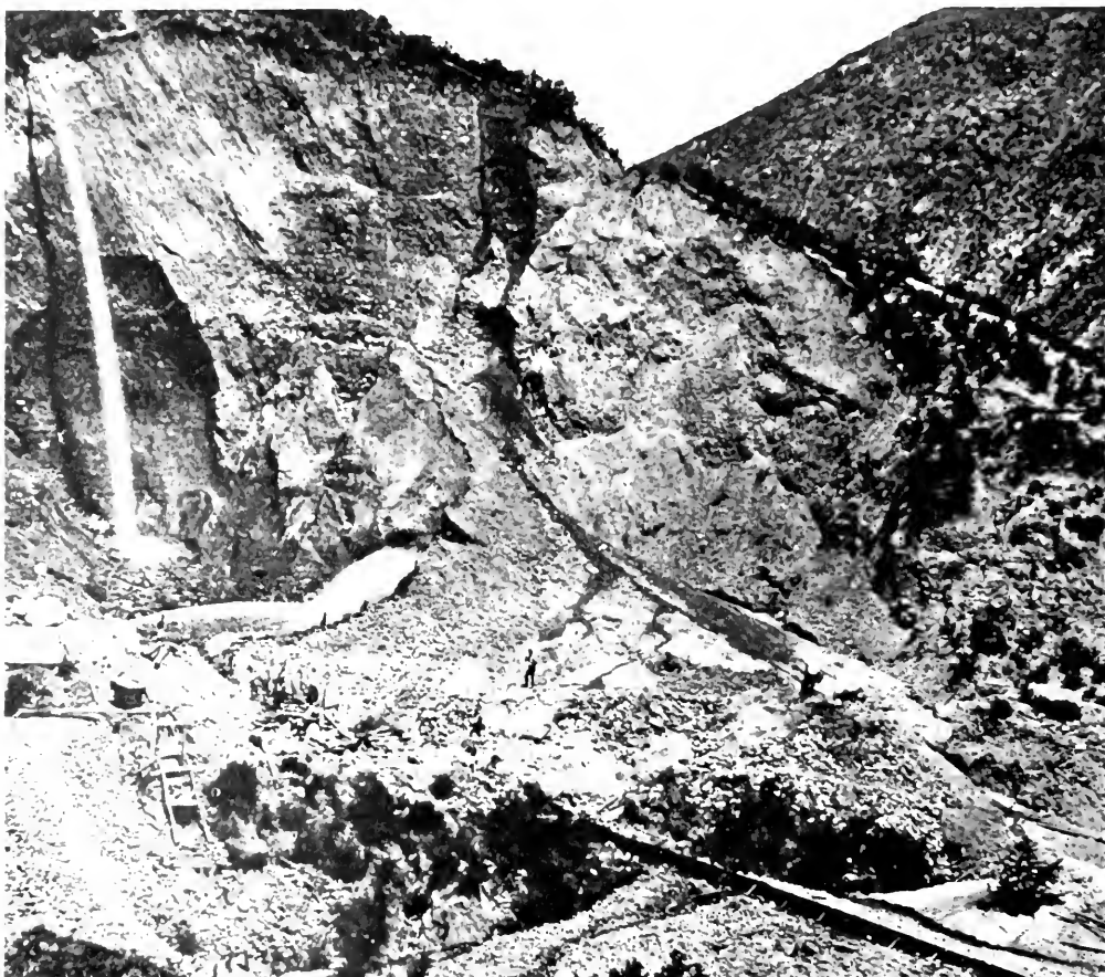
Photo 86. Lytle Creek Mine, Lytle Creek District. This photo of a hydraulic mining operation in the eastern San Gabriel Mountains, San Bernardino County, was taken in about 1894. Photo courtesy of Calif. State Library
