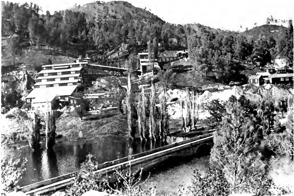
Photo 13. Carson Hill Mine and Mill, Carson Hill District. This northward view of the Calaveras County mine and large mill was taken in the 1920s. Photo courtesy of Hillcrest Studio, Angels Camp.
