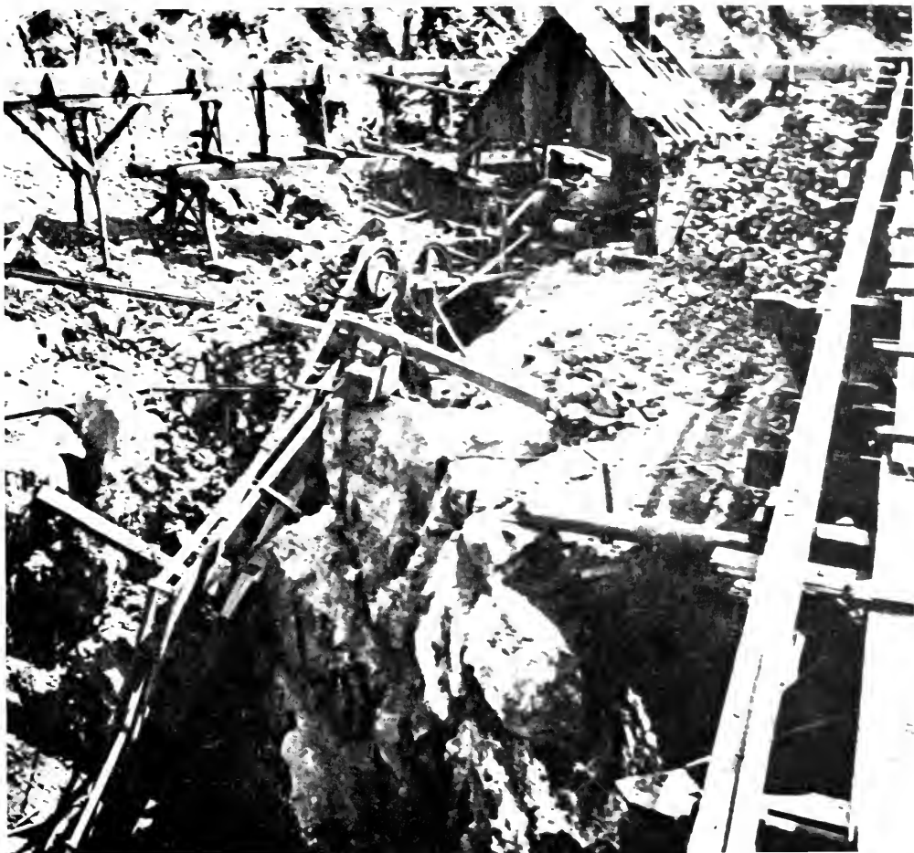
Photo 64. Early Placer Mining, Valcano District. This scene, in Valcano, Amador County, shows sluice boxes, a pump and a deep crevice in limestone bedrock.
