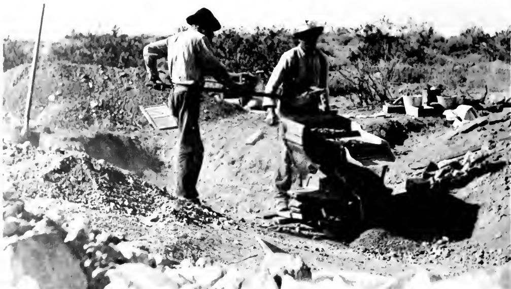
Photo 77. Dry Placer Mining, Coolgardie District. The photo was taken in San Bernardino County in the early 1900s. Photo courtesy of O. A. Russell, Yermo.
