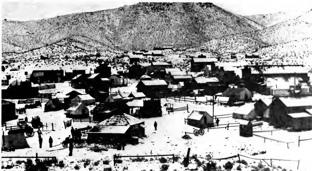
Photo 84. Town of Randsburg, Kern County. This winter view, taken in the early 1900s, looks east.
