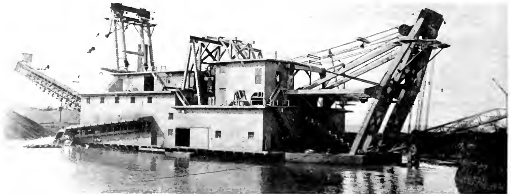
Photo 20. Natomas Company Dredge No. 9, Folsom District. This is a 1914 photo of the dredge, in Sacramento County. Photo by C. A. Waring.
