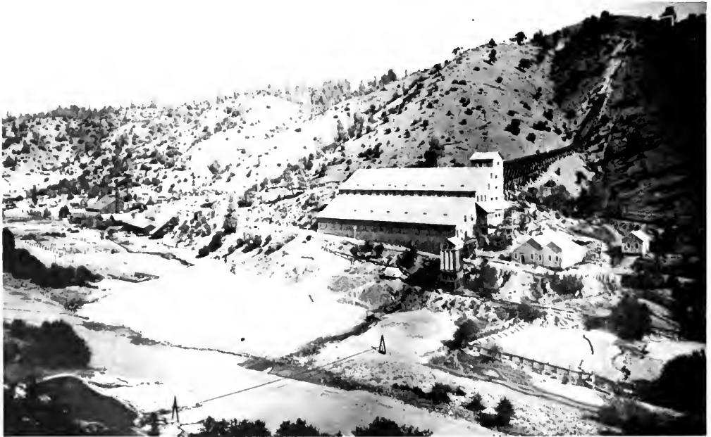
Photo 37. Eagle-Shawmut Mine, Jacksonville District. This 1914 view, looking northeast, shows the 100-stamp mill, the tramway and the tail-
