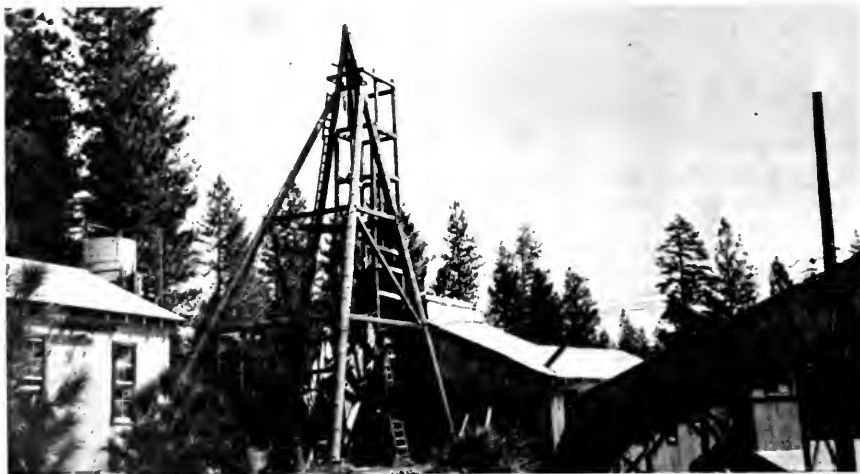
Photo 65. Belden Mine, West Point District. This 1952 view of the mine, in Amador County, looks northeast. The mine was active in the 1930s.
