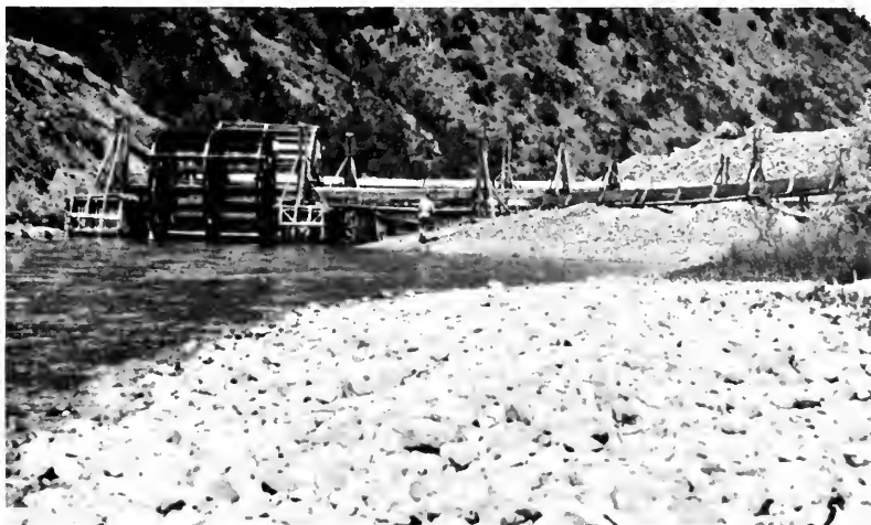
Photo 68. Placer Mine, Siskiyou County. Water wheel and flume appear in this view of a mine operated by Chinese on the Klamath River in 1933. At one time these Chinese water wheels were widely used in river mining. Photo by Olof P. Jenkins.
